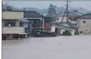
Broken houses by flood in Kagoshima Pref.
