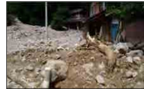
Broken houses by landslide in Nanto city
