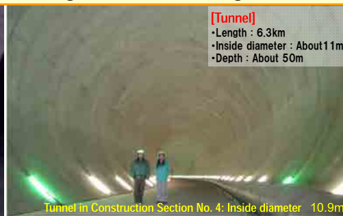
Tunnel in Construction Section No. 4: Inside diameter 10.9m
