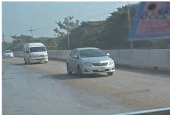
Figure F19 The flood walls by using concrete barriers; they are generally constructed along the road in flooded area in Chao Phraya River Basin
