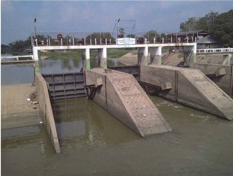
Figure F16 Wat Maneechonlakhon Regulator: The tail regulator of main drainage canal of Pasak Tai Irrigation Project, which is the important flood control structure for Muang District, Lopburi Province
