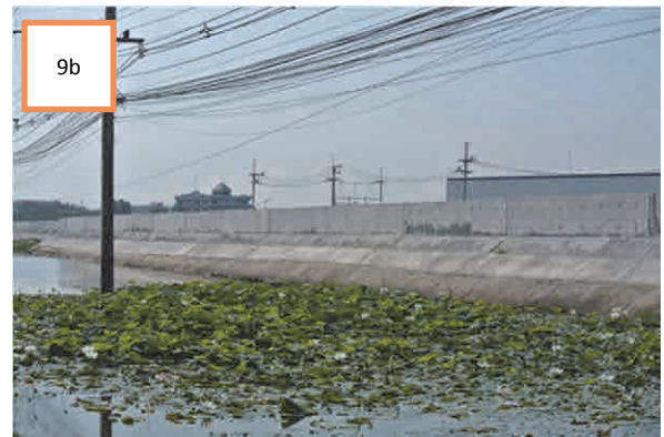
Figure F9 Flood walls at Bang Pa-In Industrial Estate, the height was added after flood in 2011, Ayutthaya Province
