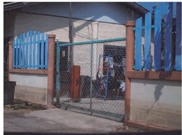
Figure F15 The flood water level in some area in Tachai Sub-district, Muang District, Chai Nat Province was smaller than beside area since the ground level is quite high due to the land fill
