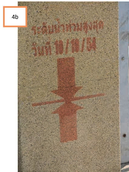
Figure F4 Some of flood marks at Sub-district Organization Office in Ayutthaya Province, in which recorded both flood peak level and time of flood peak.
