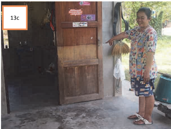
Figure F13 Water level on the walls, the best information for flood model calibration and verification in Chai Nat Province
