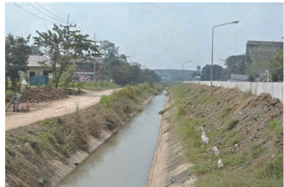
Figure F20 The back side of concrete barrier flood walls is an irrigation canal which use as a drainage canal in flood period; the households on the left hand side of the canal will obtain more flood level
