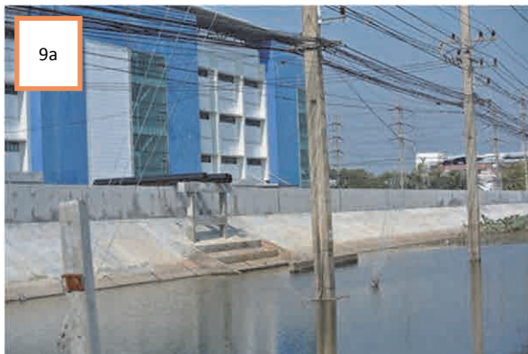
Figure F9 Flood walls at Bang Pa-In Industrial Estate, the height was added after flood in 2011, Ayutthaya Province
