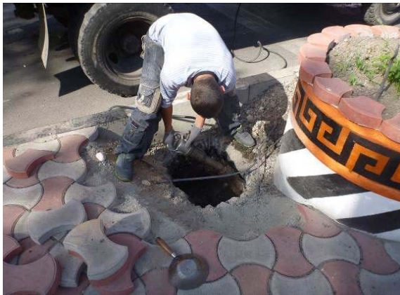
1. Excavation for Traffic Signal Pole
