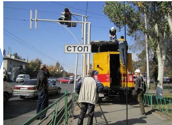
2. Installation of Traffic Signal Pole
