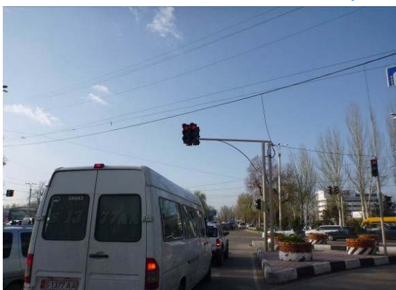
5. Installation of Lanternes
