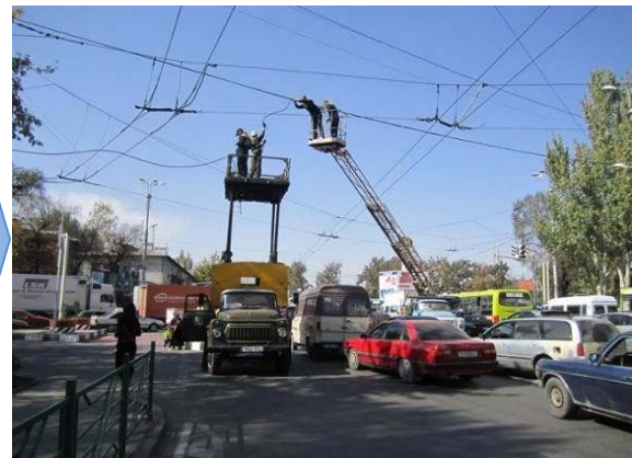
4. Wiring of Traffic Signals
