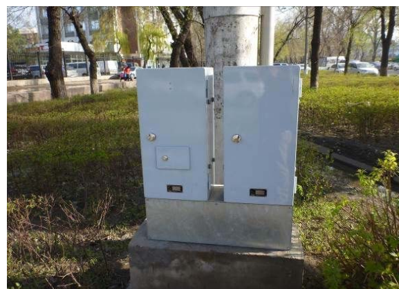
6. Installation of Local Controller
