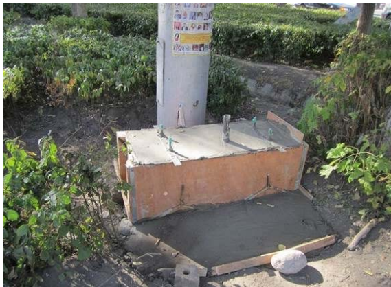
3. Foundation of Local Controller
