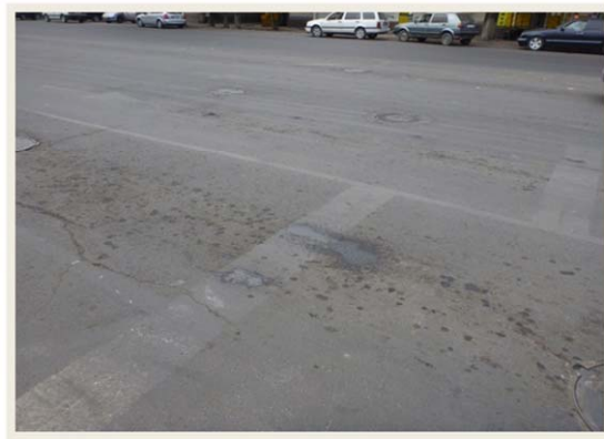
Picture A 23-1.1-11 Soiled Pavement Surface with Oil and / or Car Exhaust
