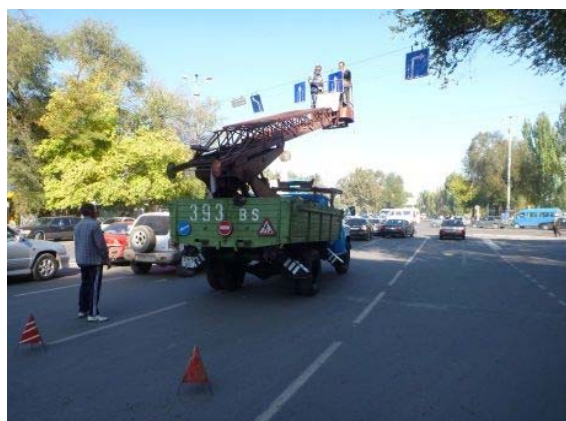
Road sign installed
