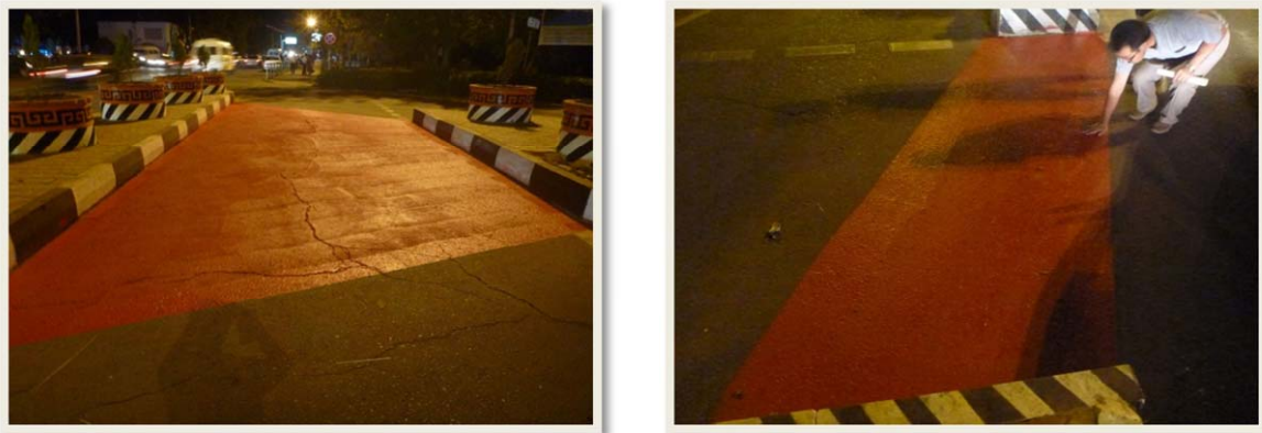
Picture A 23-1.1-13 Road Marking for Pedestrian Flow
