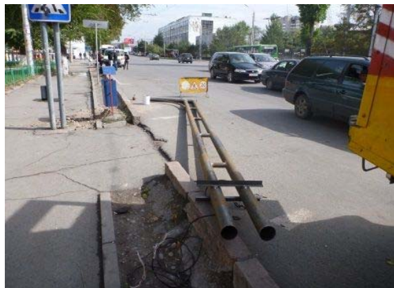
Traffic signal and the stop line relocated
