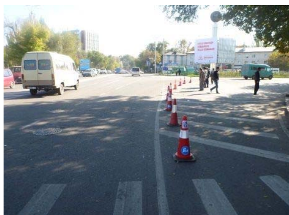
Traffic Cone installed
