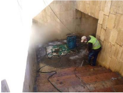
Cleaning the Pedestrian Underpass
