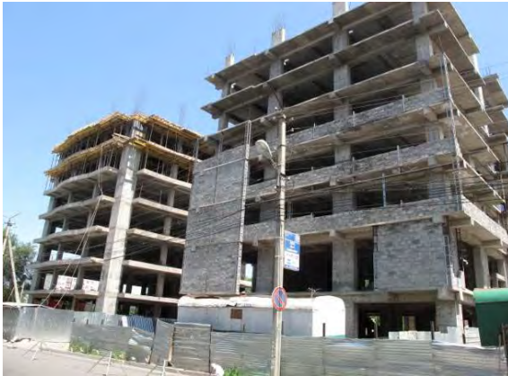
Picture 10.4-1 Construction Site in the City
