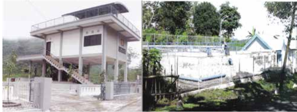
Figure 20: Flood and Landslide Monitoring Station in Lengkesse Village and Clean Water Infrastructure for the Residents of Tamalate Village, Gowa
