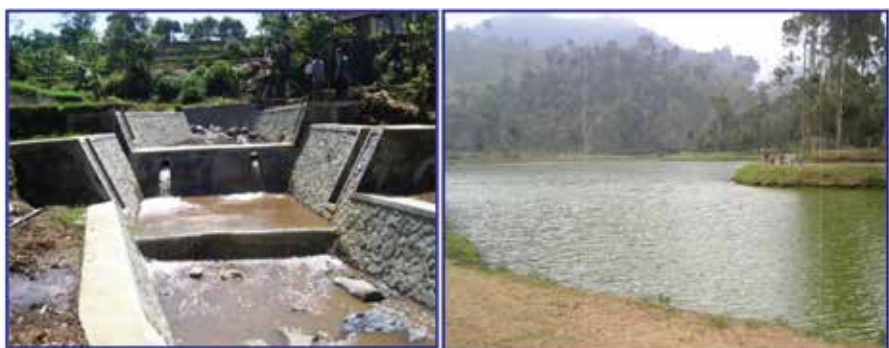
Figure 14: Check Dam Construction and Artificial Lake (situ) Rehabilitation
