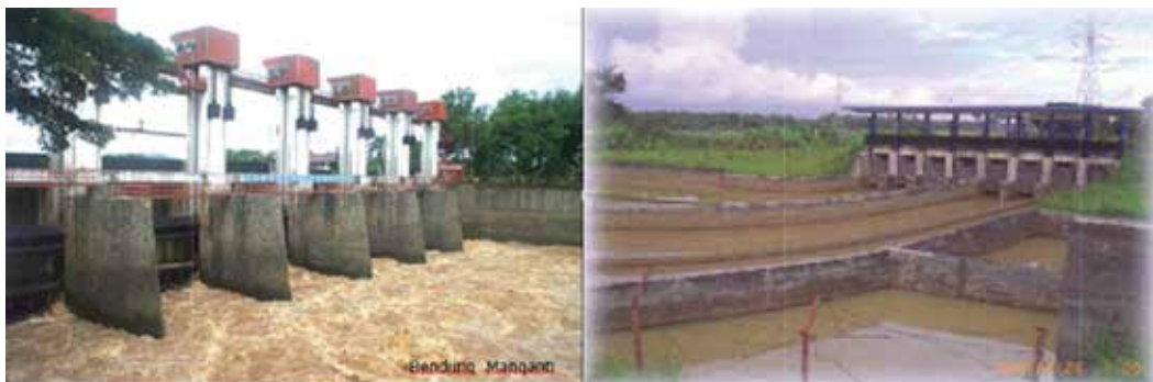
Figure 19: Manganti Weir and Cihaur-Sidareja Regulator
