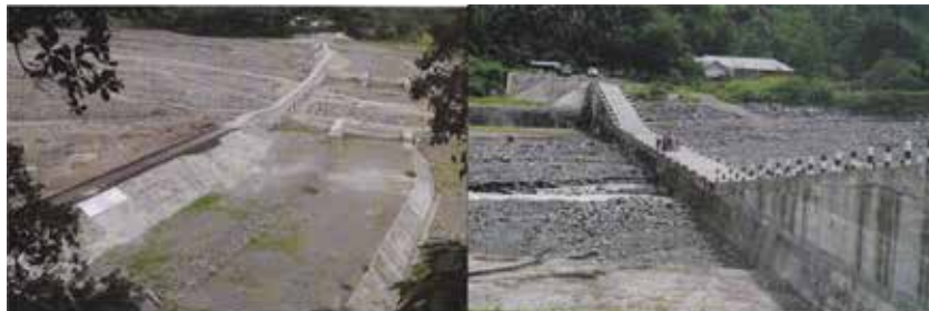
Figure 16: KD-1 and KD-2 that also function as bridges Photo by SlametWidayadi
