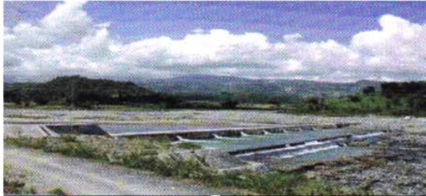
Figure 18: SP-5 before Mount Bawakaraeng landslide Source: BBWS Pompengan-Jeneberang
