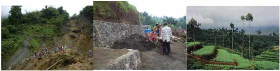
Figure 20: Landslide Management by Vegetative, Structural, and Non-Structural Methods
