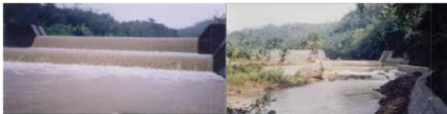
Figure 16: Goler Check-Dam and Pisitan Check-dam
