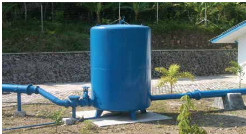
Figure 16: Raw Water Development
