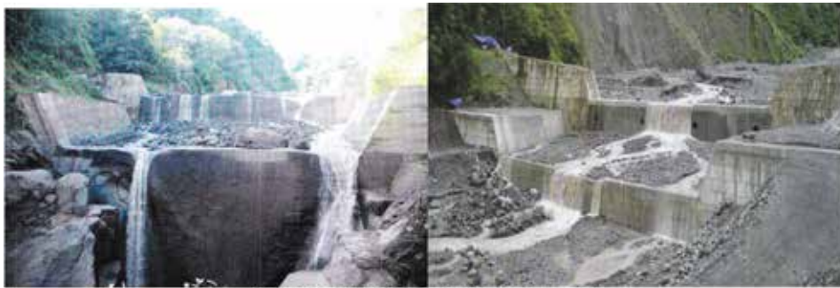
Figure 13: Sabo Dam 7-1 and 7-2
