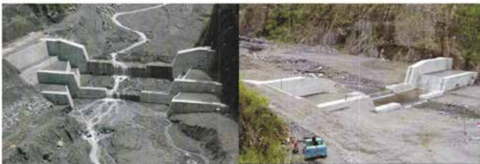
Figure 14: Sabo Dam 7-5 and 7-7
