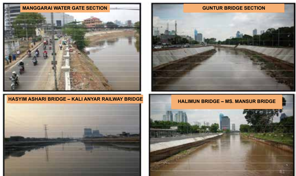
Figure 18: West Flood Canal Normalization
