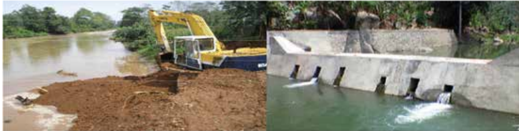
Figure 17: Flood Control Structure and River Improvement
