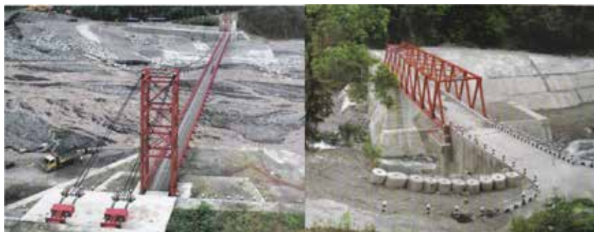
Figure 17: CD-2 and CD-3 equipped with bridges Photo by Hazama Co & YEC
