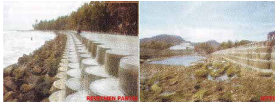
Figure 18: Revetment at Way Penet Beach and Jetty at Way Sukamaju
