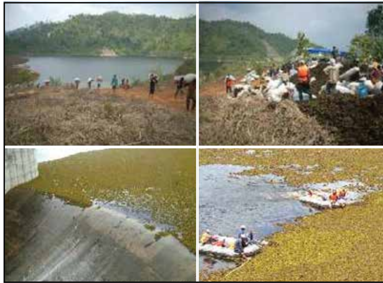
Figure 10: Over flow in Batutegi Reservoir Spillway
