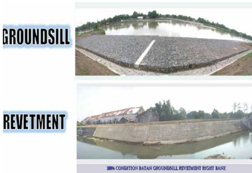
Figure 24: Groundsill and Revetment Construction
