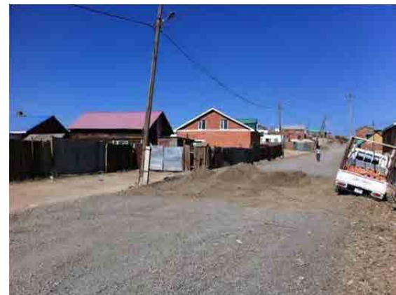
Paved road (under construction)
