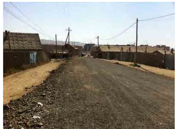
Paved road (under construction)
