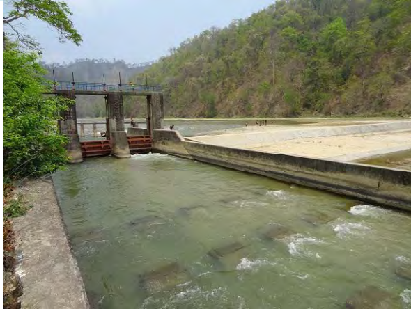
01 Kankai Headwork (Jhapa)
