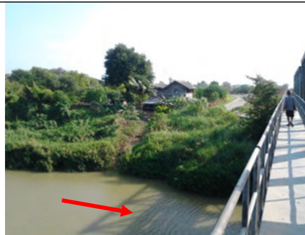
Looking Left Bank from the Railroad Bridge. (Parapet wall is installed on both right and left banks. During the 2011 Flood, the water overflowed these banks, however there was no inundation over the Railroad Bridge as elevation of the bridge abutment was high enough.)
