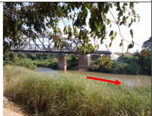
Right Bank, Looking Downstream of the Railroad Bridge
