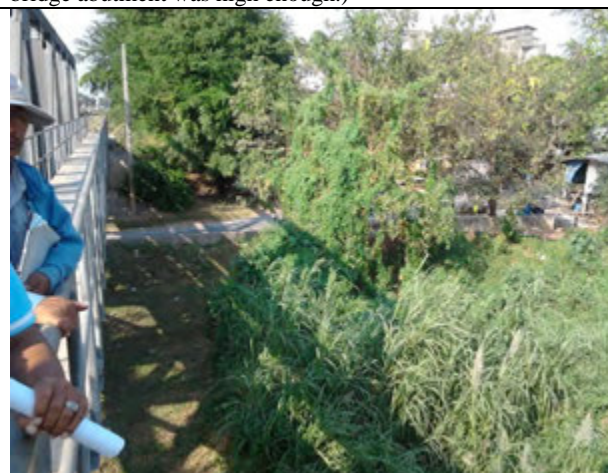
Looking at Left Bank with Parapet Wall from the Railroad Bridge. (Parapet wall is installed on right bank as well. During the 2011 Flood, the water overflowed these banks, however it is assumed that inundation over the railroad bridge was not occurred.)
