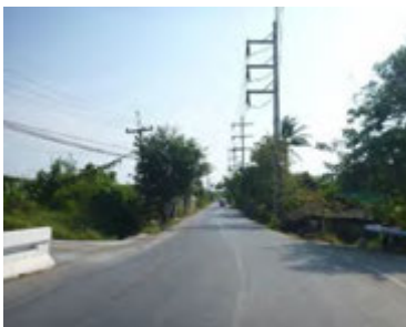
Picture L1.1.12 North of Railway
