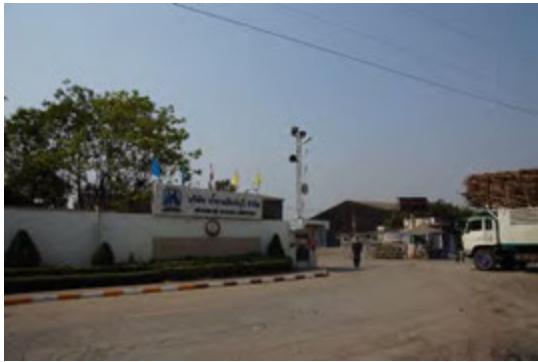
Picture L1.1.2 Sugar Factory (Inside of Secondary Dyke, Town Planning Area)
