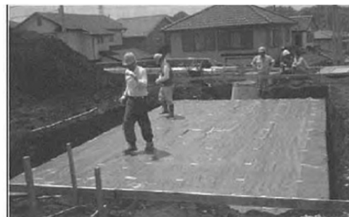
4) Placement of Sheets Work
