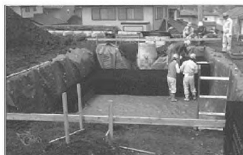
2) Assembly of Storage Structures (condition)
