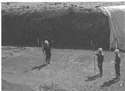
Height Control of Foundation
