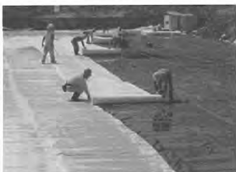
Photo 3.4-5 Placement of bottom sheets
