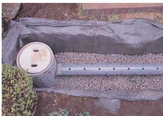
Infiltration box and Trench (Example in Japan)
