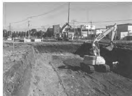
Condition of Excavation Work
