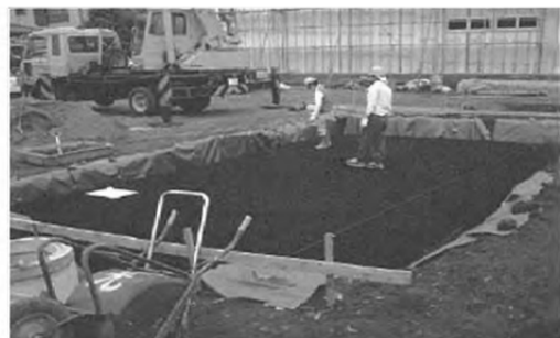
3) Assembly of Storage Structures (Completed)
