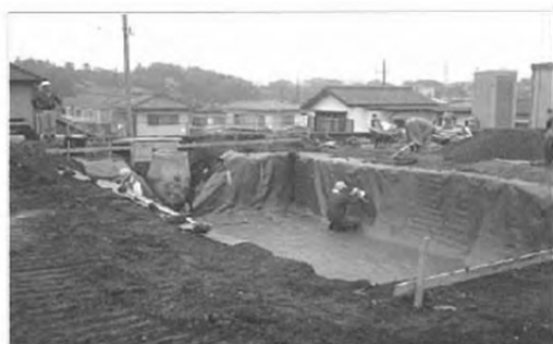
1) Excavation Work, Placement of Sheets work
