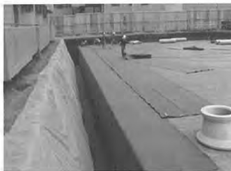
Photo 3.4-6 Placement of top sheets
