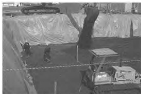
Crushed stones in the foundation
