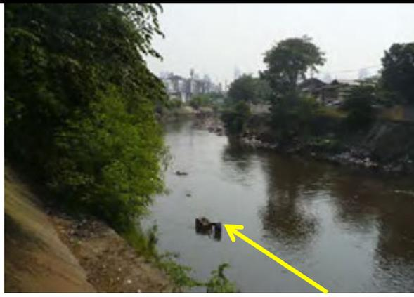
Figure 8.4-1 Deposition of Sediment, Garbage in River Channel at Downstream of Manggarai Point
