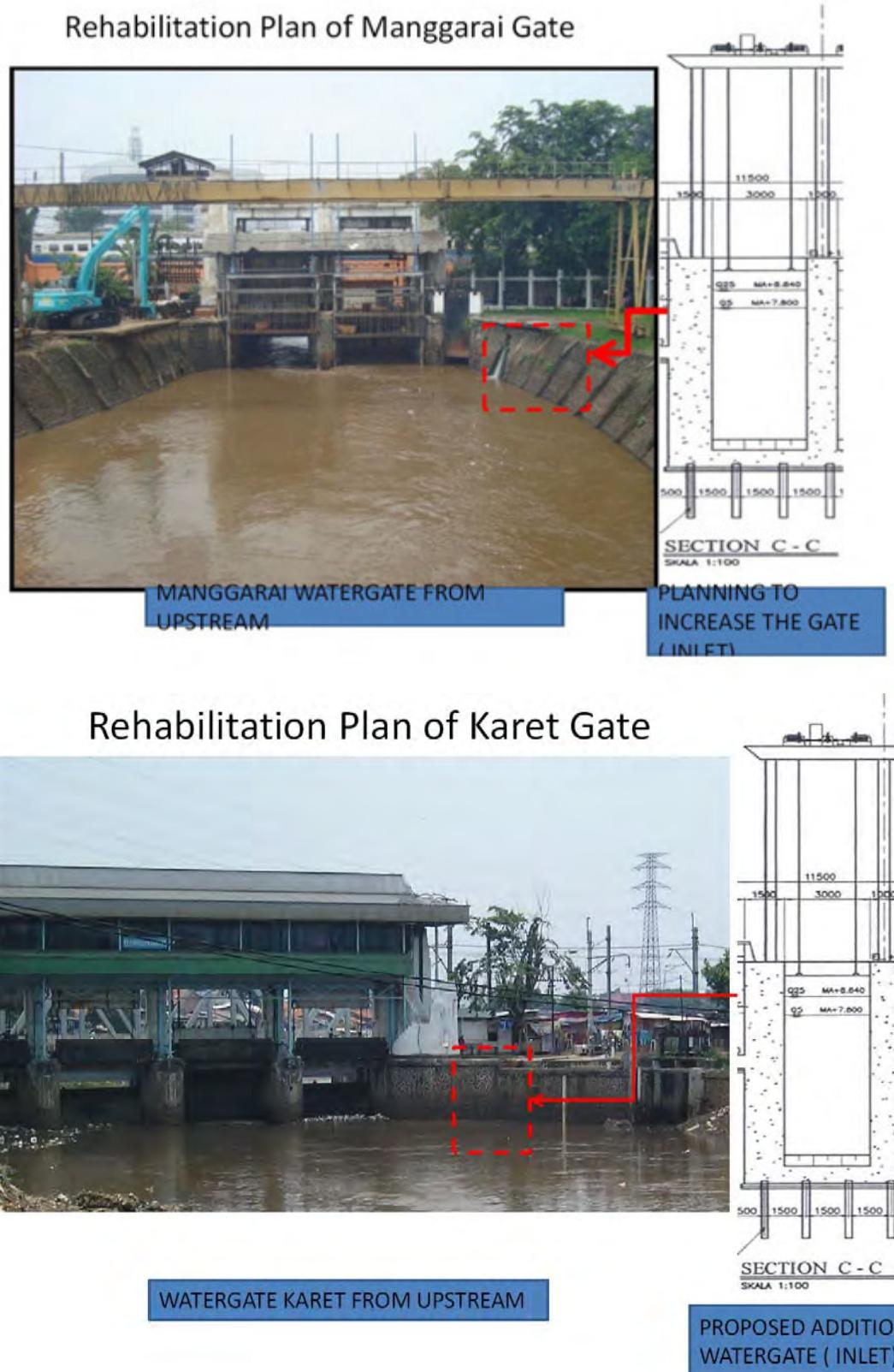
**Figure 1.5-9      Image of Rehabilitation Plan of Manggarai Gate and Karet Weir**
