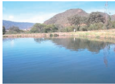
Rehabilitated wastewater treatment ponds in the Municipality of Comarapa, Bolivia
