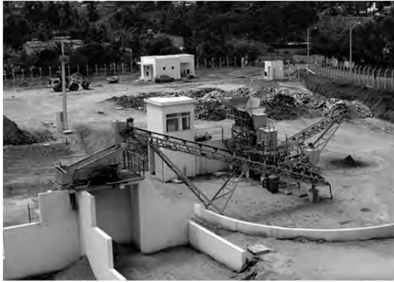
(4) Fixed waste recycling plant
