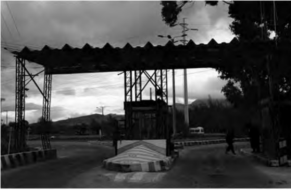
Access area to RSDJ
