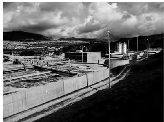
Treatment Plant for Percolated Liquids
