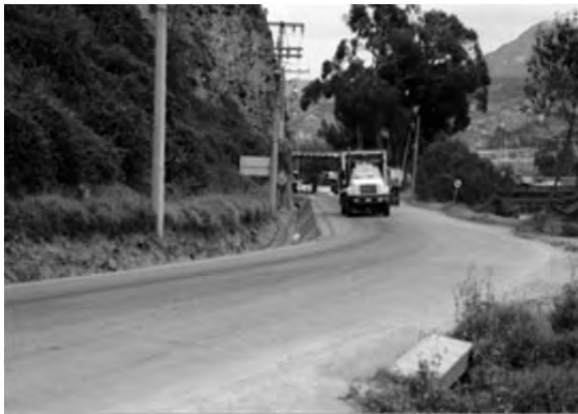
Paved access roads 1
