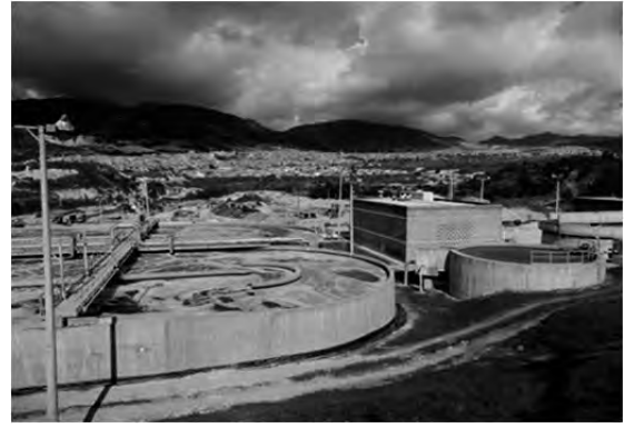
Treatment Plant for Percolated Liquids
