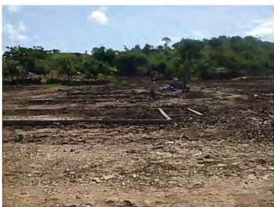
[Wesoru] – 1. Construction newly Started in April
