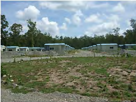
[Uma Boco-Fehuk Krin] – 1. Completed 126 House Units (while water has not been provided yet)
