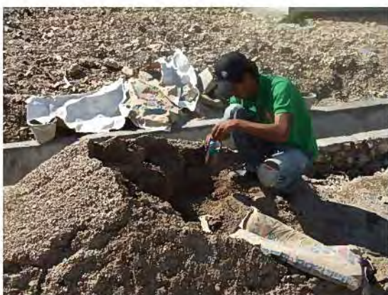
[Mehara] – 3. Sands Sampled by Engineer (Replacement directed by Engineer)
