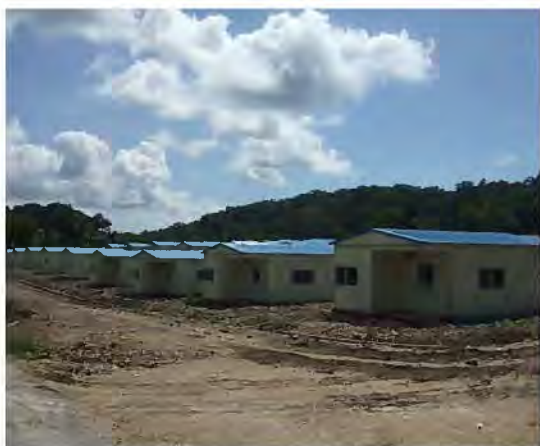
[Mehara] -1. Roads & Channels under Construction
