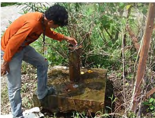
[Aubeon-Buburlaran] – 3. Existing Borehole without Pump set (Considered as possible source)
