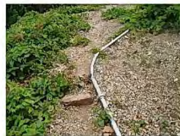
photo-12: bending without bend-joint
