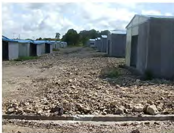
[Mehara] – 2. Drainage Channels under Construction
