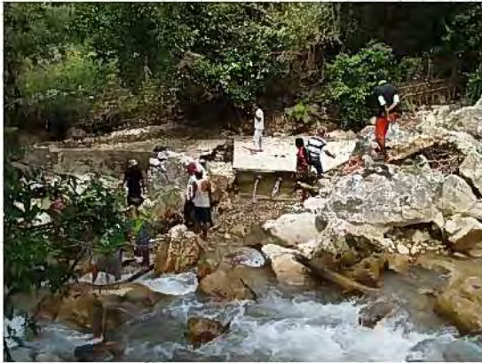
photo-1: Overall view of the Intake facilities and Transmission pipe
