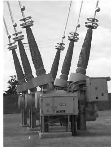
SF6 Gas Circuit Breakers
