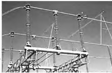
Horizontally Mounted Double-Break Switch.
