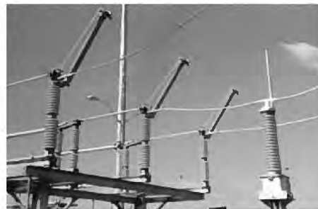
Horizontally Mounted Vertical-Break Interrupter
