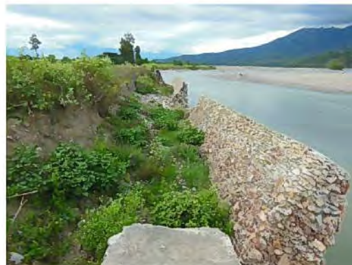
100m upstream from Bridge
