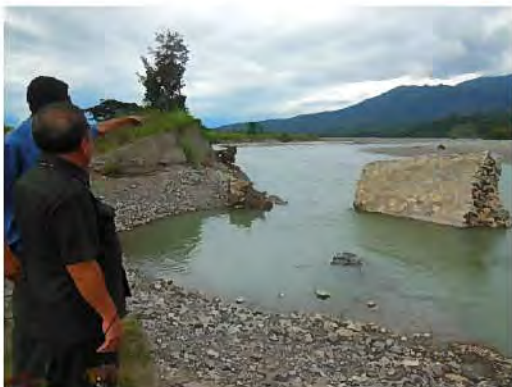
200m upstream from Bridge
