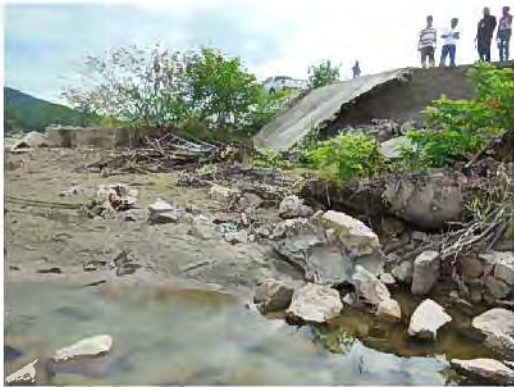
Damaged Revetment
