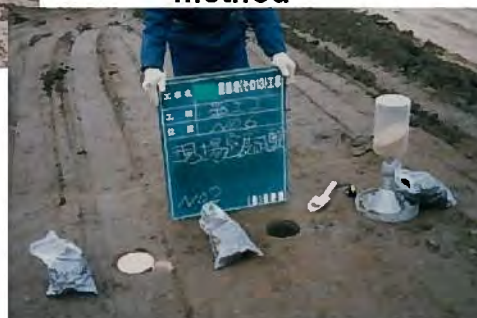
Soil density by the sand replacement method
