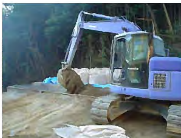
Mix of cement
