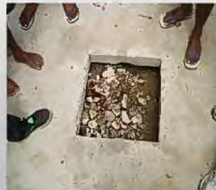
Construction without partition wall
