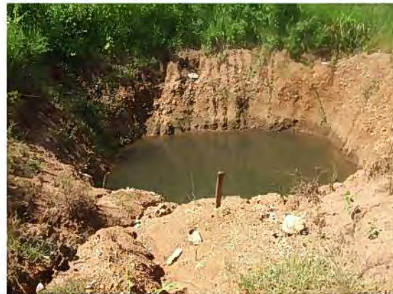
[SP4] – 2. Dug Well under Construction
