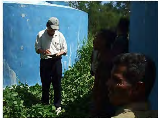
[Uma Boco-Fehuk Krin] – 4. Storage Reservoir No.2 located on a hill (50m 3 x 2 basins), high enough to supply water to the project site by gravity
