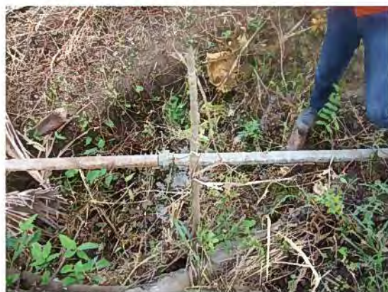
[F-FDTL] - 4. Nebee iha we matak(raw water) transmisaun too F-FDTL F-FDTL (iha diameter, GSP 4km x 3")
