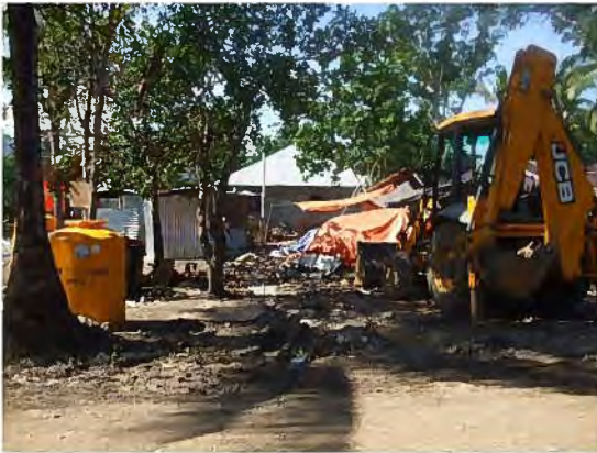
[Wesoru] – 3. Backhoe for Earthwork
