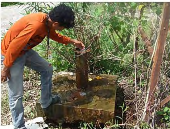
[Aubeon-Buburlaran] – 3. Existing Borehole without Pump set (Considered as possible source)
