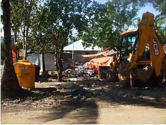
[Wesoru] – 3. Backhoe for Earthwork
