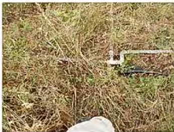
photo-11: complex jointing
