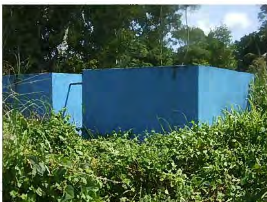
[Uma Boco-Fehuk Krin] – 3. Reservador lubu ida (Ground Storage) No.1 ba sidade (basia 20m 3 x 2)
