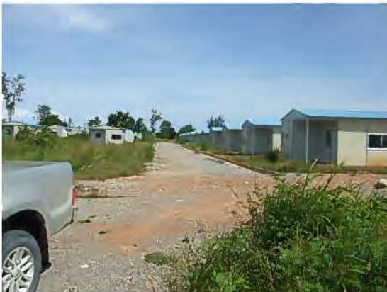
[SP4] – 1. Overview of Project Site
