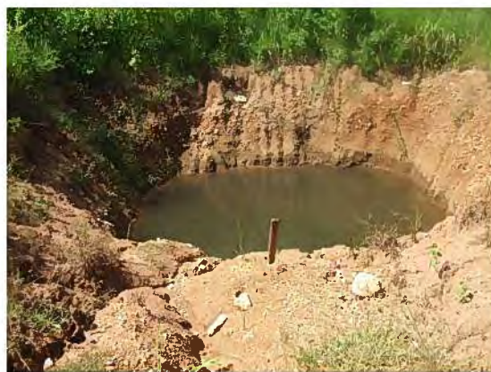
[SP4] – 2. Konstrusaun kee bee posu halao hela( Dug Well under Construction)
