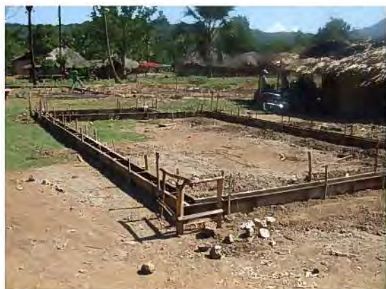
[Wesoru] – 2. Foundation with Reinforcement
