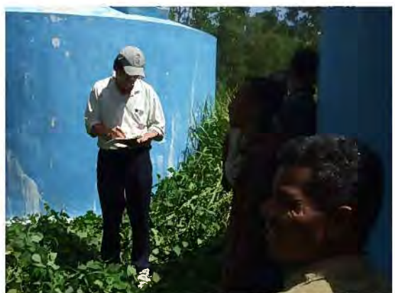
[Uma Boco-Fehuk Krin] – 4. Storage Reservador No.2 aloka iha foho leten (basia 50m 3 x 2) projektu husi graviti (gravity) suficiente fornese bee .
