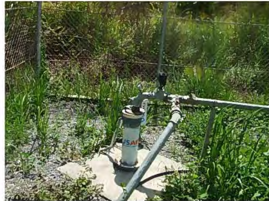
[Uma Boco-Fehuk Krin] – 2. Borehole Constructed by USAID in 2010 (62m in depth, not in operation because of a lack of gov. budget for operation)
