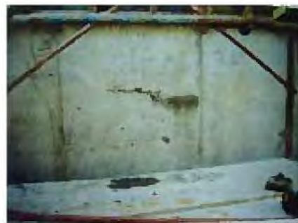
Cold Joints/sedimentasaun didin
