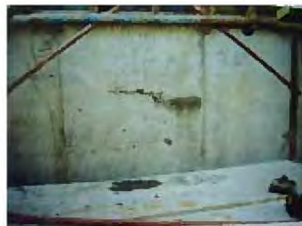
Cold Joints/sendid dingin
