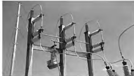
Vertically Mounted Vertical-Break Switch
