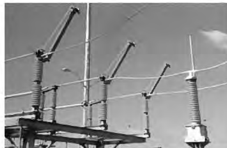
Horizontally Mounted Vertical-Break Interrupter
