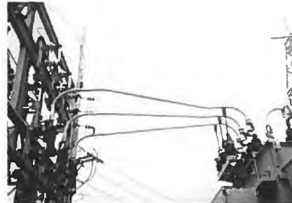
Hook Stick Switches on Structure at Termination of Bus from Transformer
