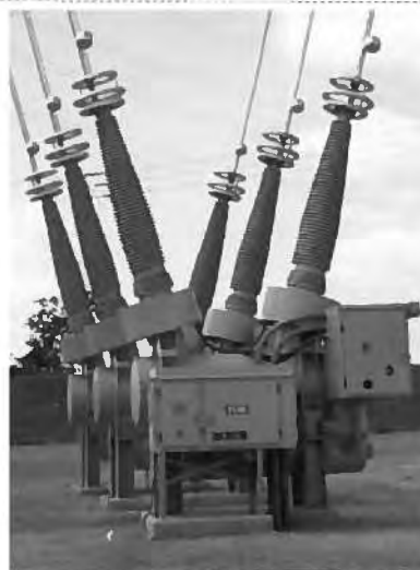
SF6 Gas Circuit Breakers
