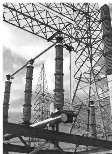
Horizontally Mounted Double Break Switch with Grounding Switch
