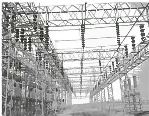
Suspension Insulator
