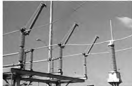
Horizontally Mounted Vertical-Break Interrupter
