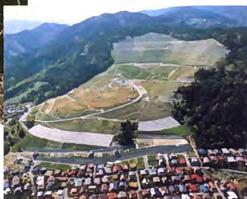
After Completion of Prevention Works
