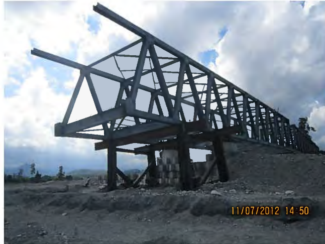
AYASA BR. Erected using temporary supports and crane
