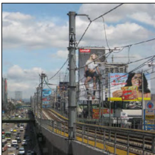
Photo 2-2 H beam pole system of NEP OCS
