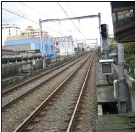
Photo 2-1 Portal beam system of Original OCS
