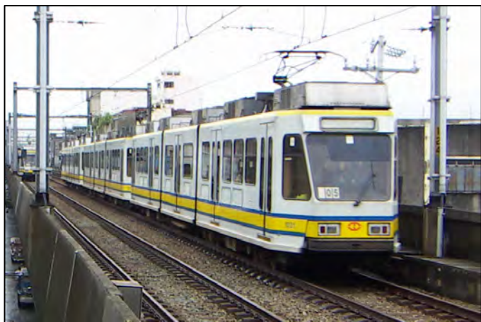
Figure 3-2 First Generation Train (Air Conditioned)
