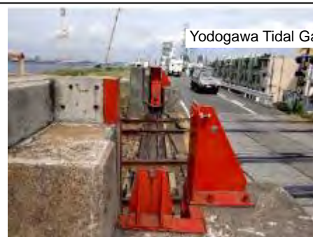
Figure: Example of a tidal gate (railway)
