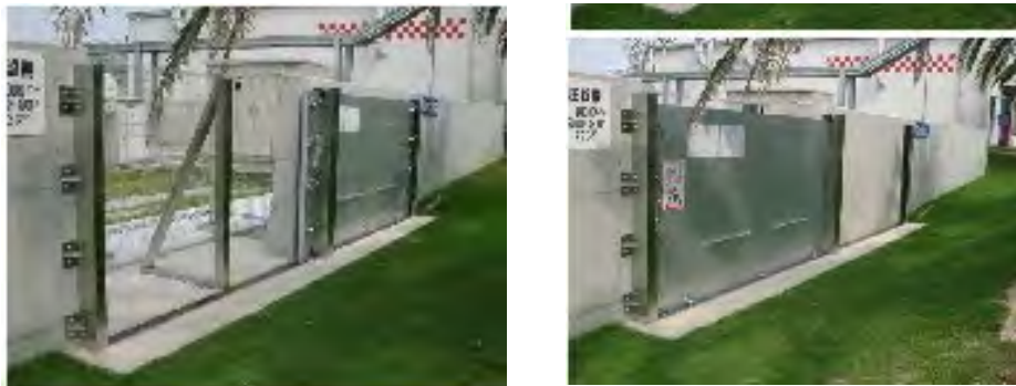
Figure: Example of cut-off wall (electrical facility)
