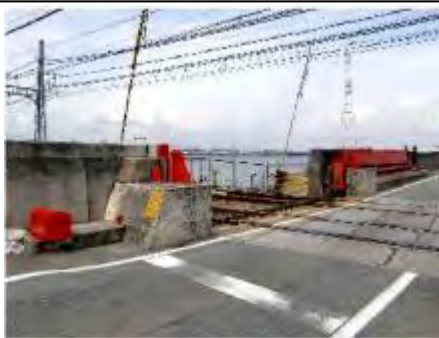
Figure: Example of a tidal gate (railway)
