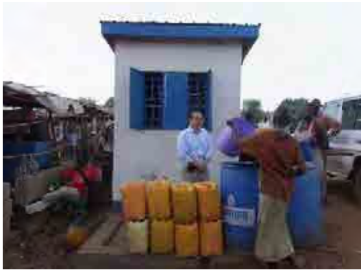
Public tap stand (Before installing a 2000 m3 tank)
