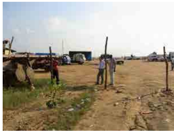
Training for Supervision of Fence Installation
