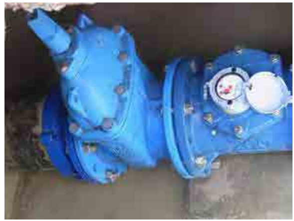
Installation of flow meter
