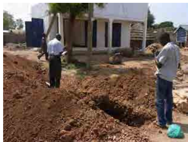
Training for distribution and transmission 2 (Recording of new service pipe installation)
