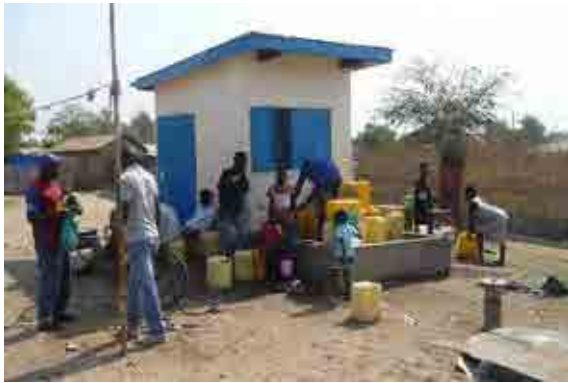
Construction of pilot public tap stand for trial operation
