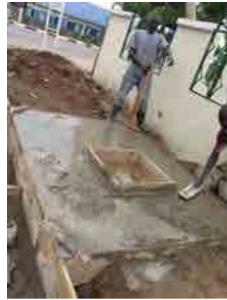
Construction flow meter pit
