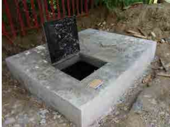
Construction of flow meter pit
