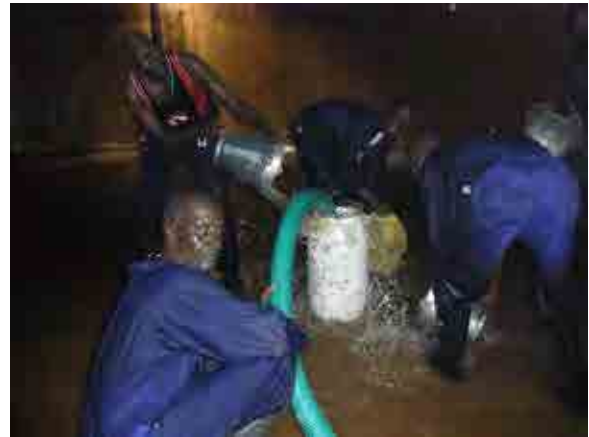
Pumping water out from the clear water tank
