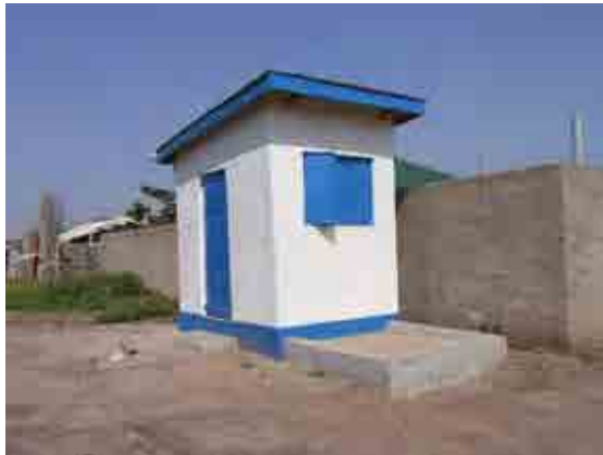
Construction of pilot public tap stand for trial operation
