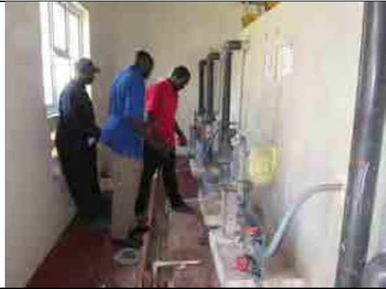
Installation of chlorine injectors
