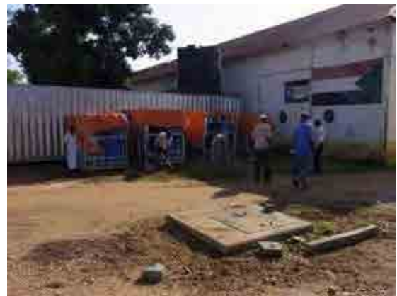
Cleaning in the purification plant
