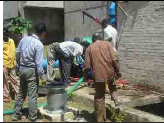
Installation of electromagnetic flow meter
