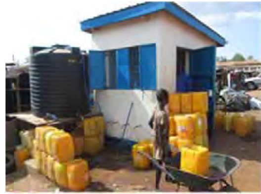
Public tap stand (After installing a 2000 m3 tank)
