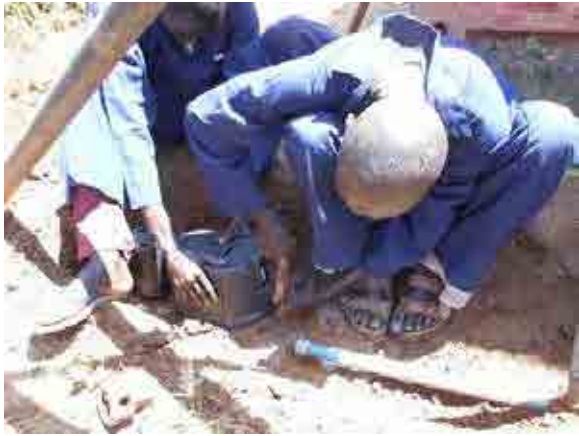
Installation of Customer Meter (Test Meter Field)
