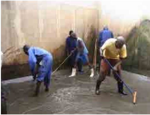
Training for water purification (Cleaning of raw water tank)
