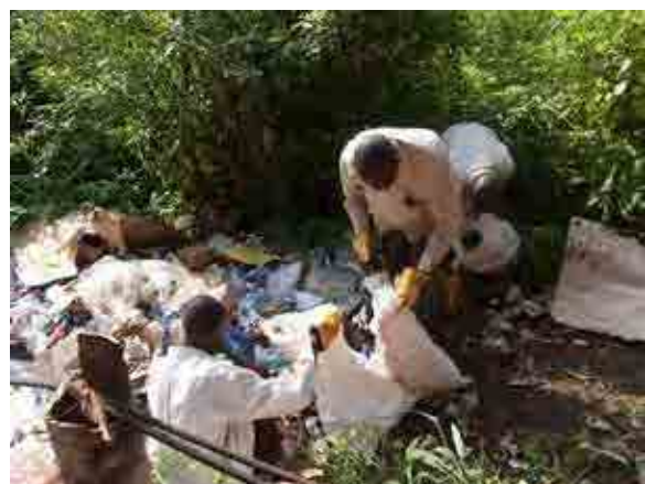
Cleaning in the purification plant (2)
