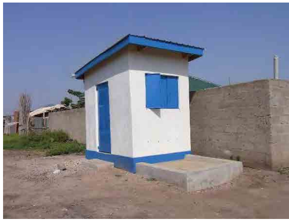
Construction of pilot public tap stand for trial operation
