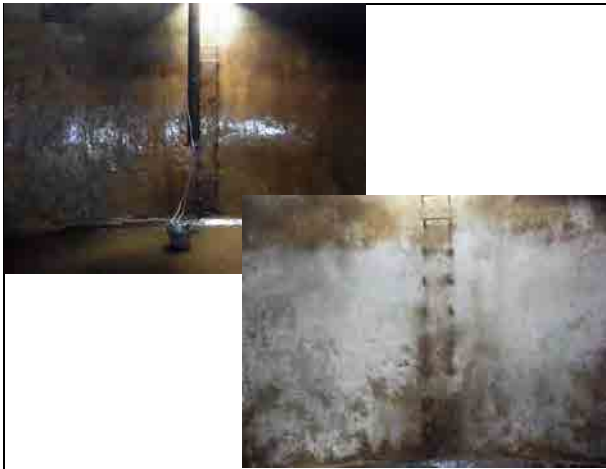
Cleaning activities for the clear water tank Before and after the tank inside
