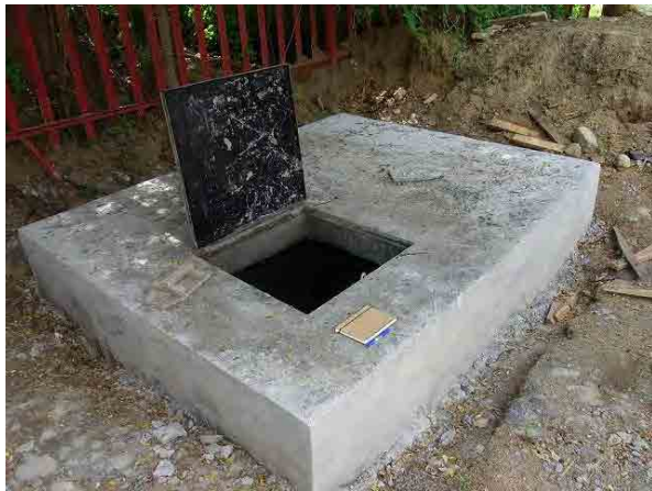
Construction of flow meter pit
