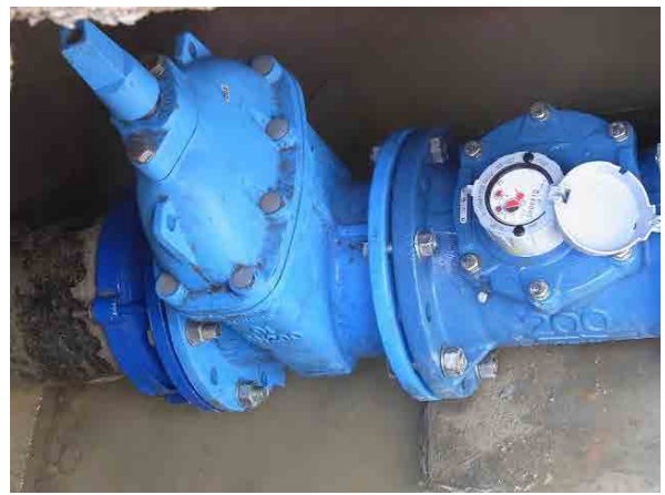
Installation of flow meter
