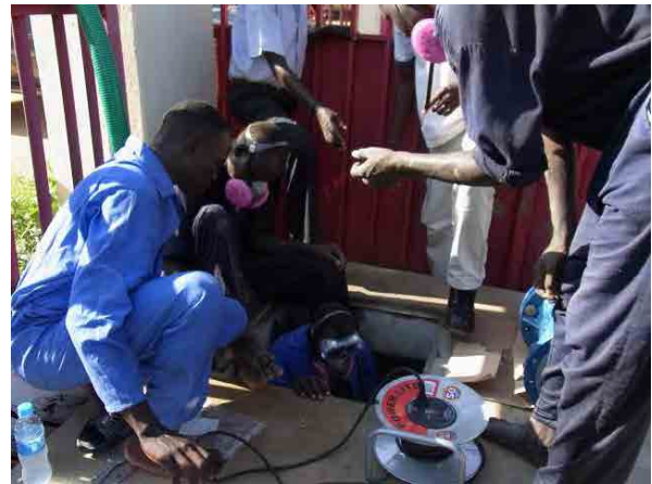
Training for distribution and transmission 2 (Protection in cutting asbestos cement pipe)
