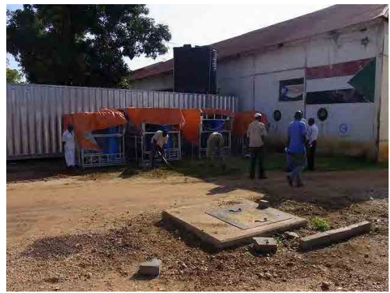
Cleaning in the purification plant
