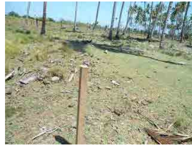
Downstream of Drainage Canal 2
