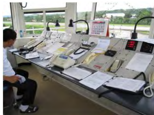
FSS Console inside of Tower
