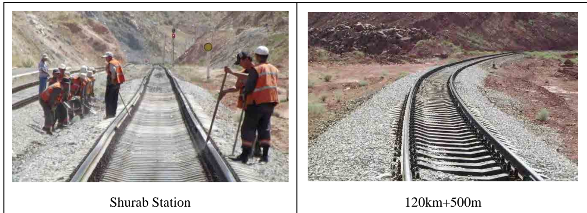
[Fig. 2-16] Location with Replaced Ballast
