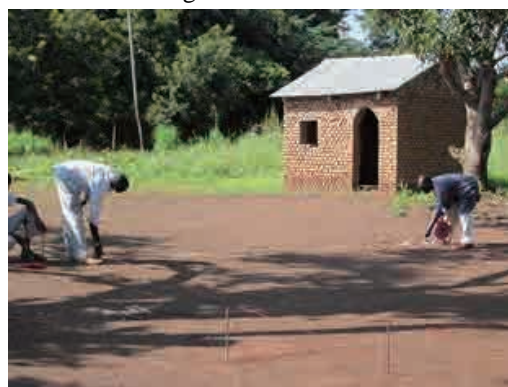
Construction course: Survey work
