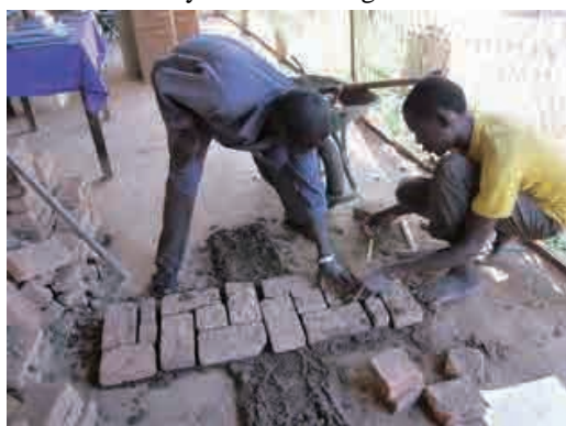
Construction course: Brick masonry
