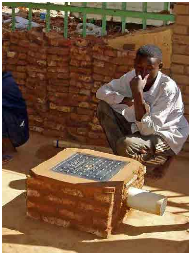
Building Course in Omdurman VTC
