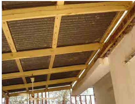
Roof of Khartoum 3 VTC (A/C Section)
