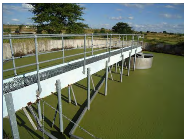
Picture 13 Final Sedimentation Tank
