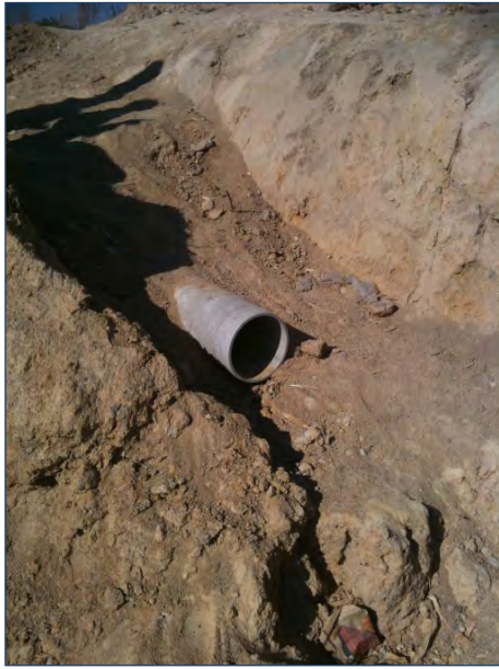
Picture 16: New Sewer Pipes Installed by AWA Funds
