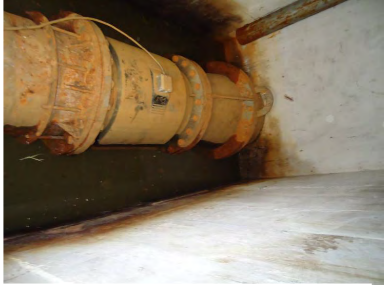
Photo A5.1.1 Inside of Meter Pit There is almost no strait pipe
