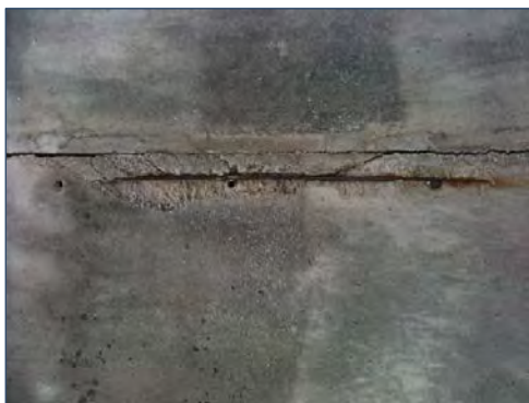
Picture 6: Cracks on the 1975 Trickling Filter Wall
