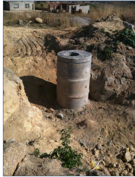
Picture 17: New Sewer MH Installed by AWA Funds
