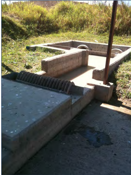
Picture 22: Vertical Chamber in Pump Station III
