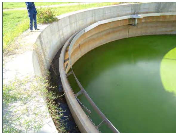
Picture 10: Primary Sedimentation Tank
