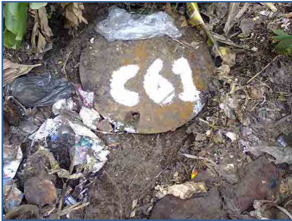
Photo 7.2.6 Debris in the Manhole because of Close Rubbish Dumps
