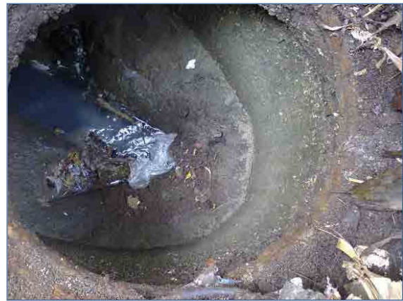
Photo 7.2.6 Debris in the Manhole because of Close Rubbish Dumps
