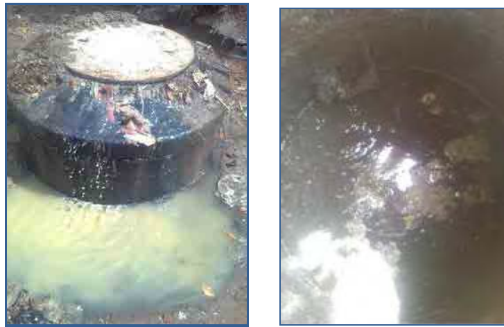
Photo 7.2.1 Overflowing Manholes
