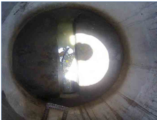
Subsurface inflow through rings
