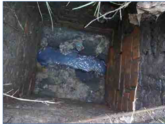
Photo 7.2.7 Debris in Manholes because of Improper Lid and Use of Newspapers by Residents
