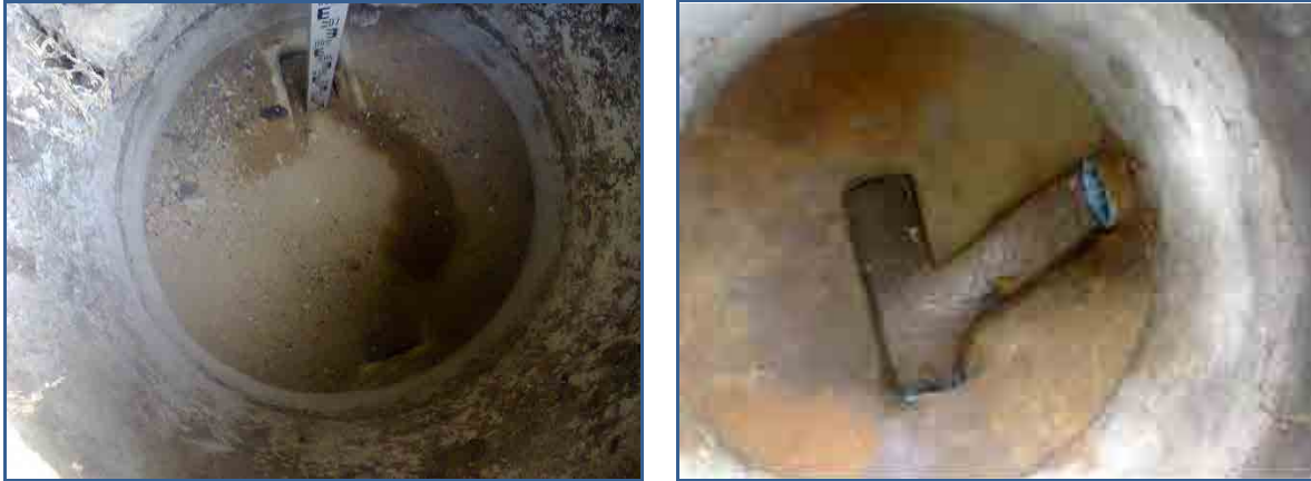
Photo 7.2.5 Sand on Benching and Base Channel
