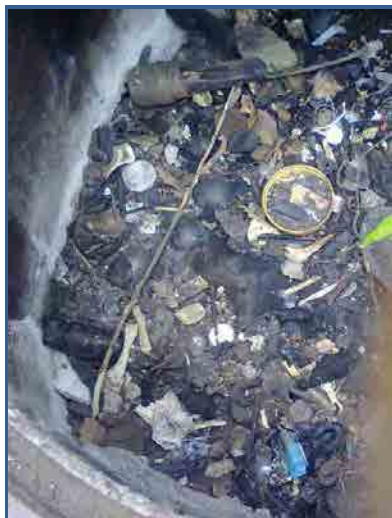
Containers, bottles, soil Broken stove plate Photo 7.2.8 Manholes in Residential Stands Used as Rubbish Dumps
