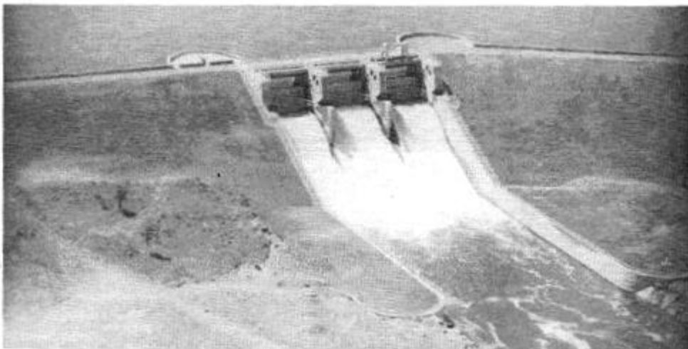
Photo 2.4.2 Spillway of Manyame Dam
