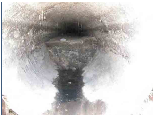
Photo 4.2.1 Sand Deposit in the Sewers in Chitungwiza
