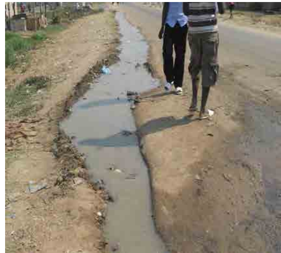
Photo 2.5.2 Sewage from burst pipes often finds its way to open canals posing health threats to the residents.
