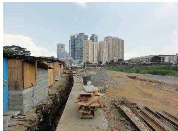
Cleared riverside and new parapet in Santolan area
