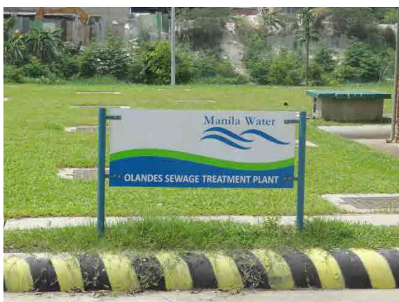
Sewerage plant built by Manila Water
