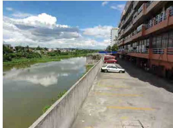
Private protection walls are commonly be seen, and they sometimes obstruct river flow
