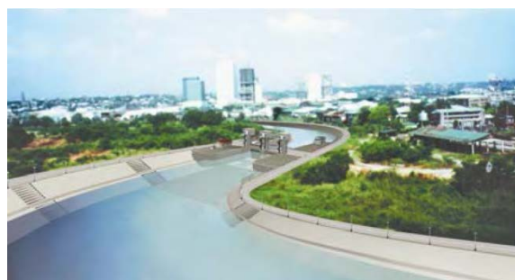
Bird's view from upstream side
