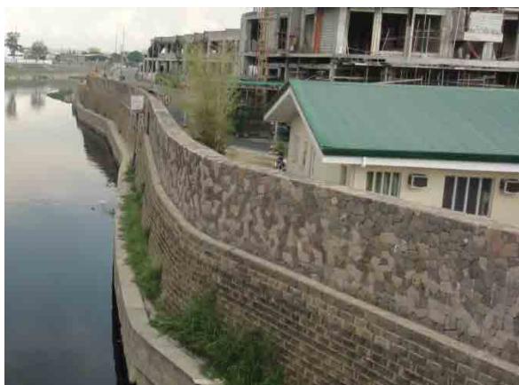
Circulo Verde's river wall at upstream side of Rosario Weir
