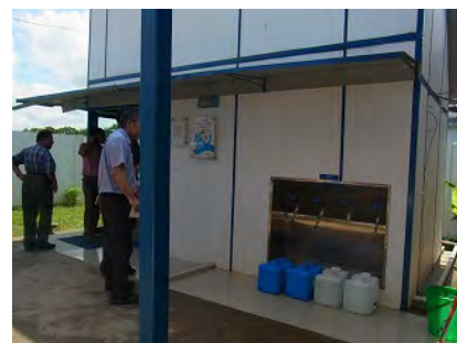
WaterHealth Centre of A.K. Khan WaterHealth Ltd. in Raojan, Chittagong Division
