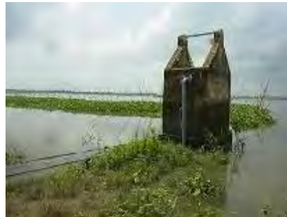
Water Intake Tower of the WTP
