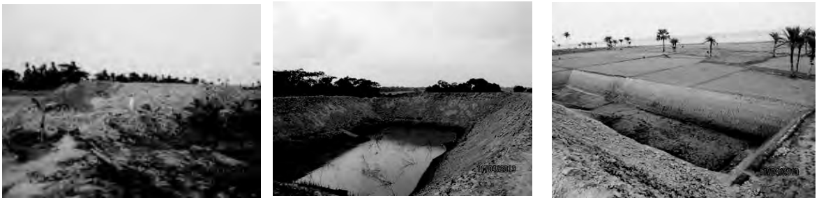
Killa in Lord Harding union under construction
