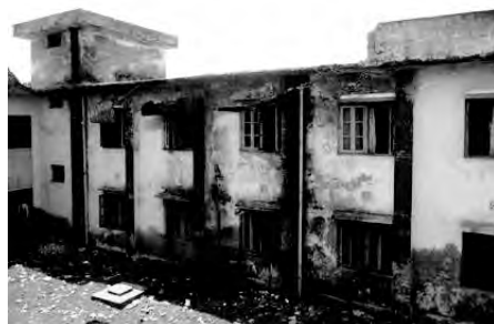
Mongla upozila parishad building
