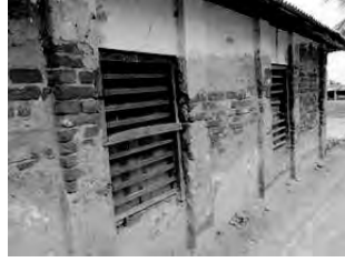
Salinity and brick structure
