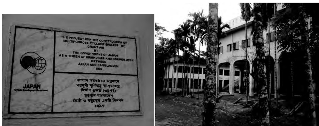
Pictures: Japan Govt. funded cyclone shelter in Purba char bata.
