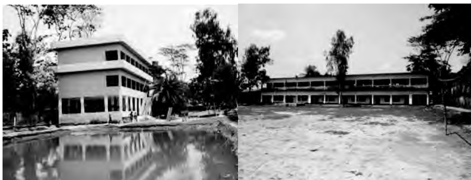
Cyclone shelters at charduanti union
