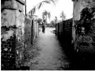
Salinity and brick structure
