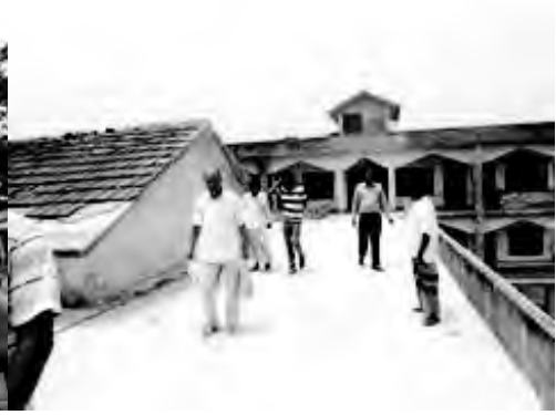
Union parishad cum cyclone shelter
