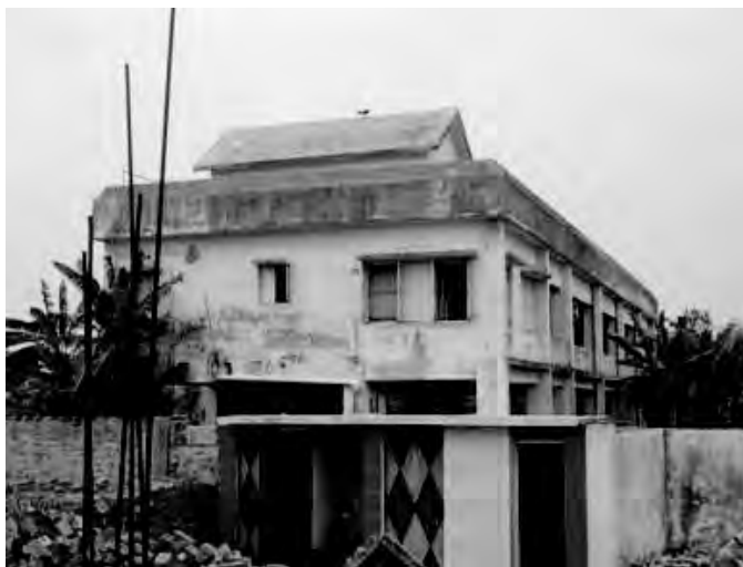
Picture: Project CDSF funded cyclone shelter in Nizhum Dwip.
