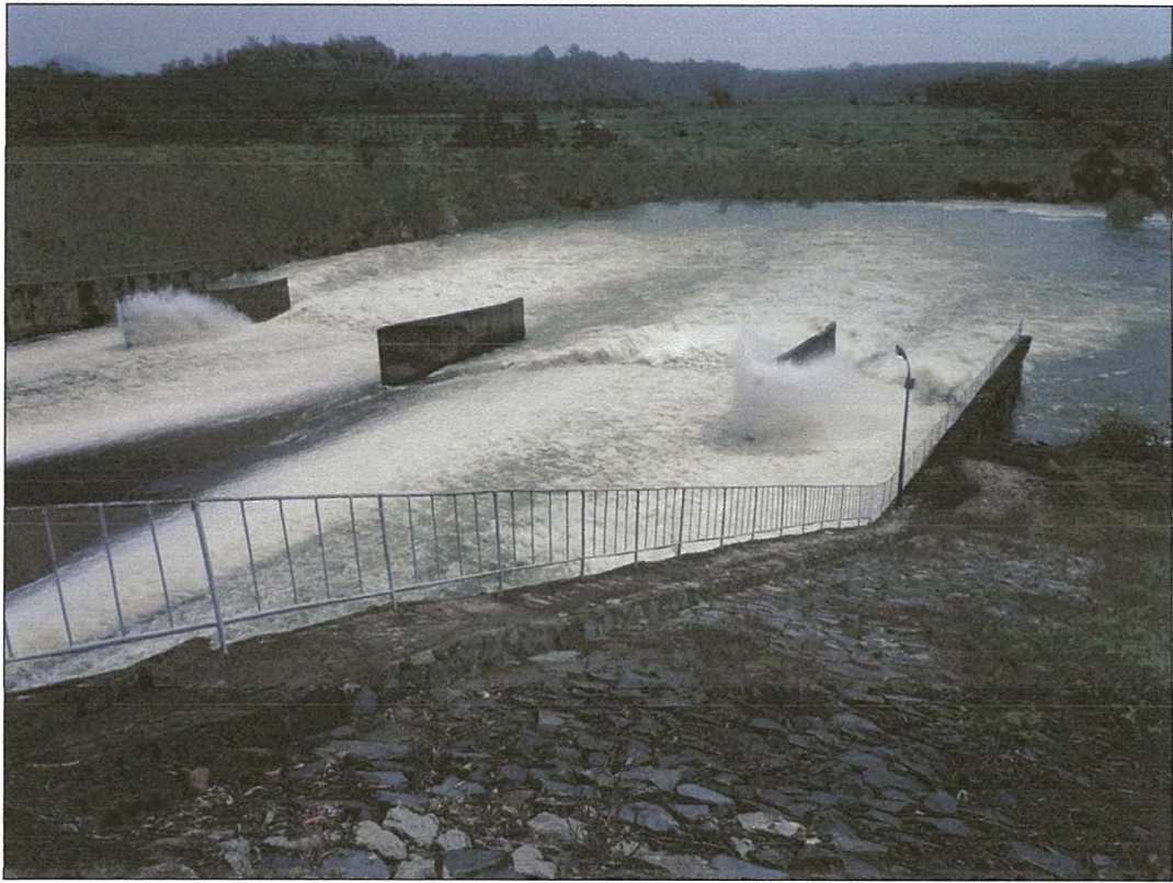
Dau Tieng Irrigation dam – Dau Tieng District – Binh Duong Province
