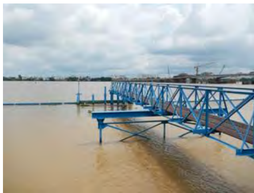
Hoa An Intake Pump N=6 (1)
