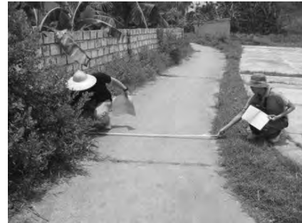
Concrete paved road (w=2.1m)
