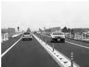
Center poles in expressway in Japan
