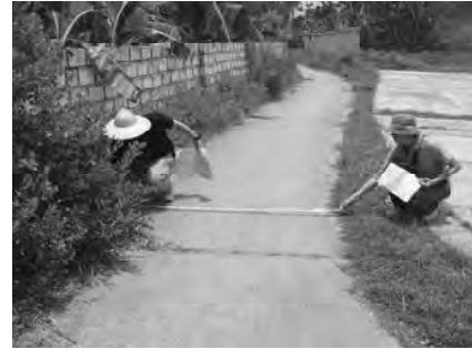
Concrete paved road (w=2.1m)
