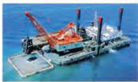
Dredging frame with silt curtain
