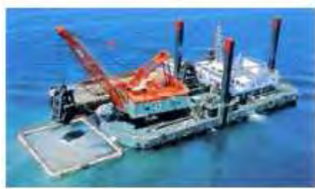
Dredging frame with silt curtain
