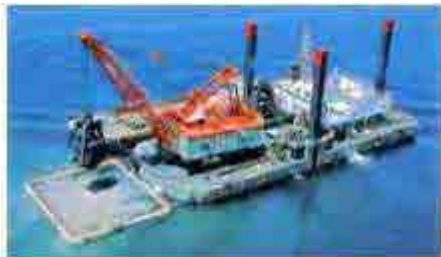
Dredging frame with silt curtain
