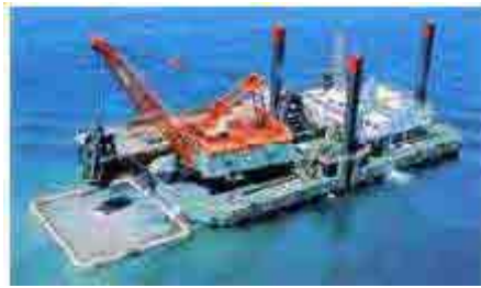
Dredging frame with silt curtain (silt curtain frame)
