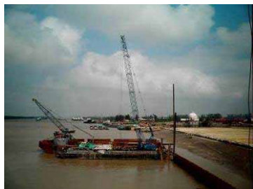
Crane Barge 50t
