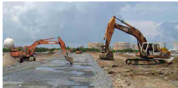
Excavator ( 0.7\text{ m}^3 )
