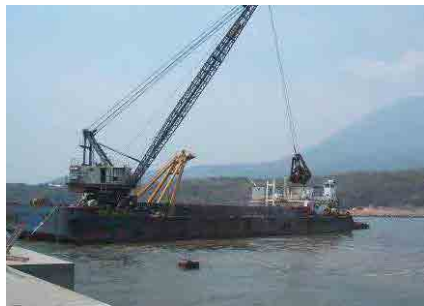
Grab Dredger (5.0m 3 )
