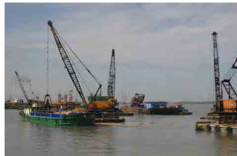
Grab Dredger (2.0m 3 )
