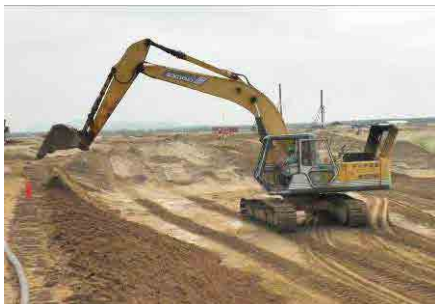
Excavator ( 0.7\text{ m}^3 )
