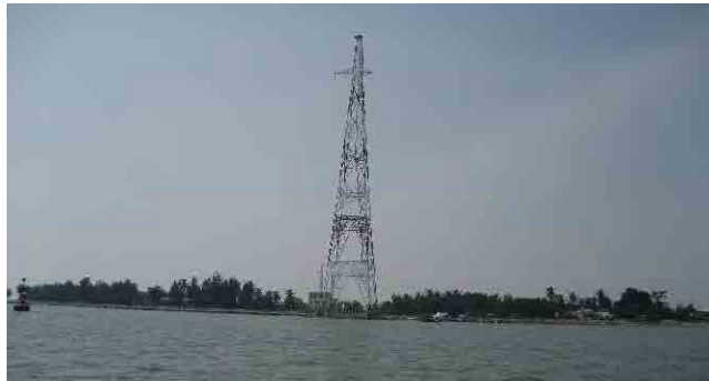
Figure 10.1.1 High Voltage Power Line Tower
