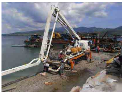
Concrete Pump Truck (60m 3 /h)
