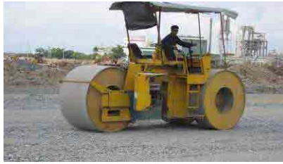
Compaction Roller (4t)
